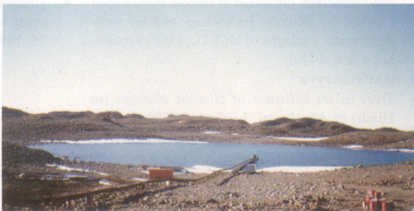
Part of Zub Lake showing pipe line supplying water to Maitri Station
